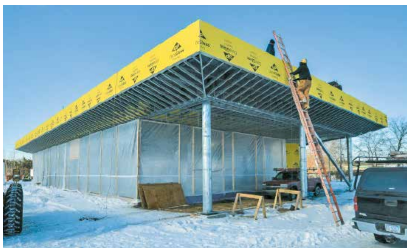
Capital Area Multimodal Gateway, operated by CATA, under construction.
