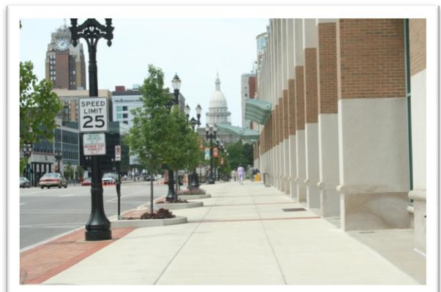
The Lansing Center's renovated façade removed the front driveway and replaced it with additional square footage, access to the street, and other treatments to make an attractive, accessible, and safe area for pedestrians - Lansing, MI
