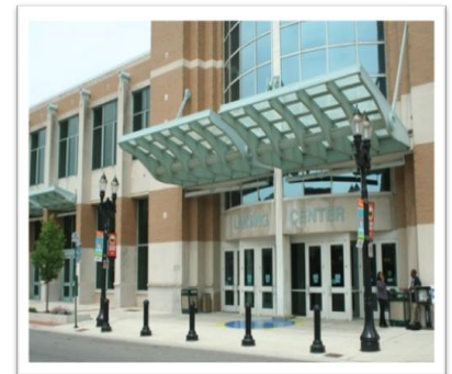
Lansing Center, Lansing, MI
