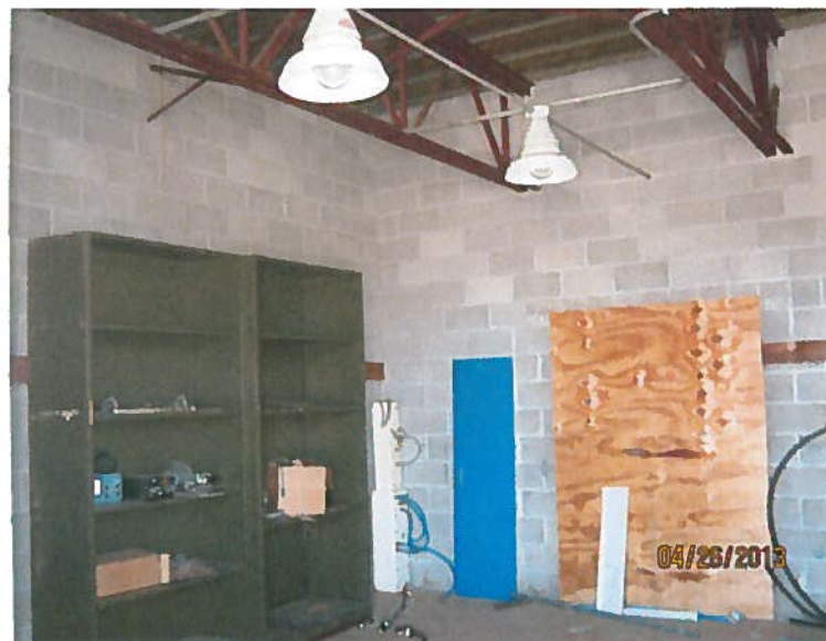
Photograph No. 10 Compact Fluorescent Light Bulbs Storage Building A
