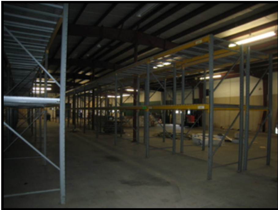
Photograph No. 15 View of Building 4 – interior
