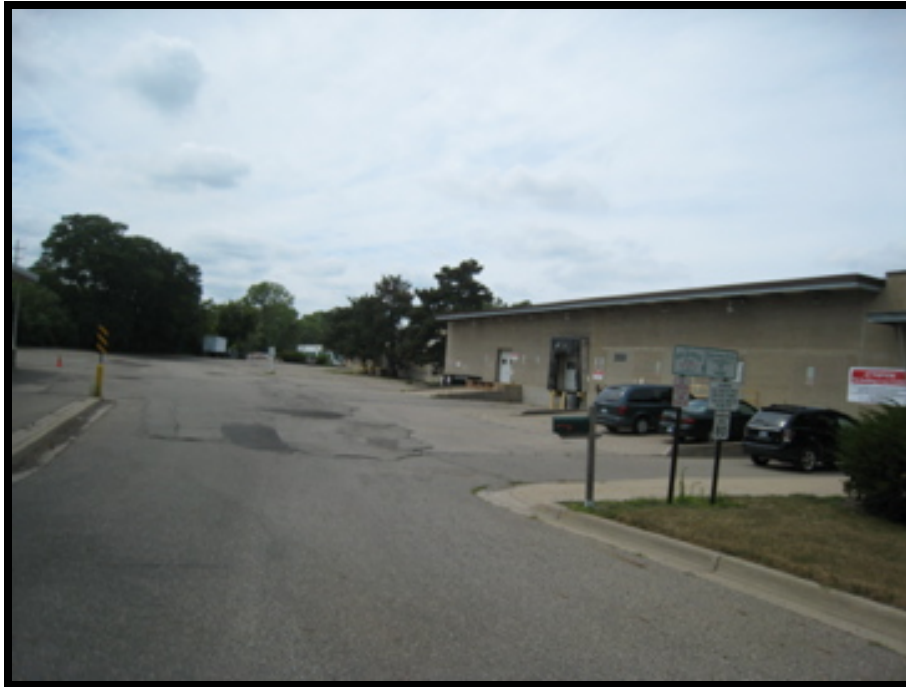
Photograph No. 5 View of subject property – Building 2 – facing west
