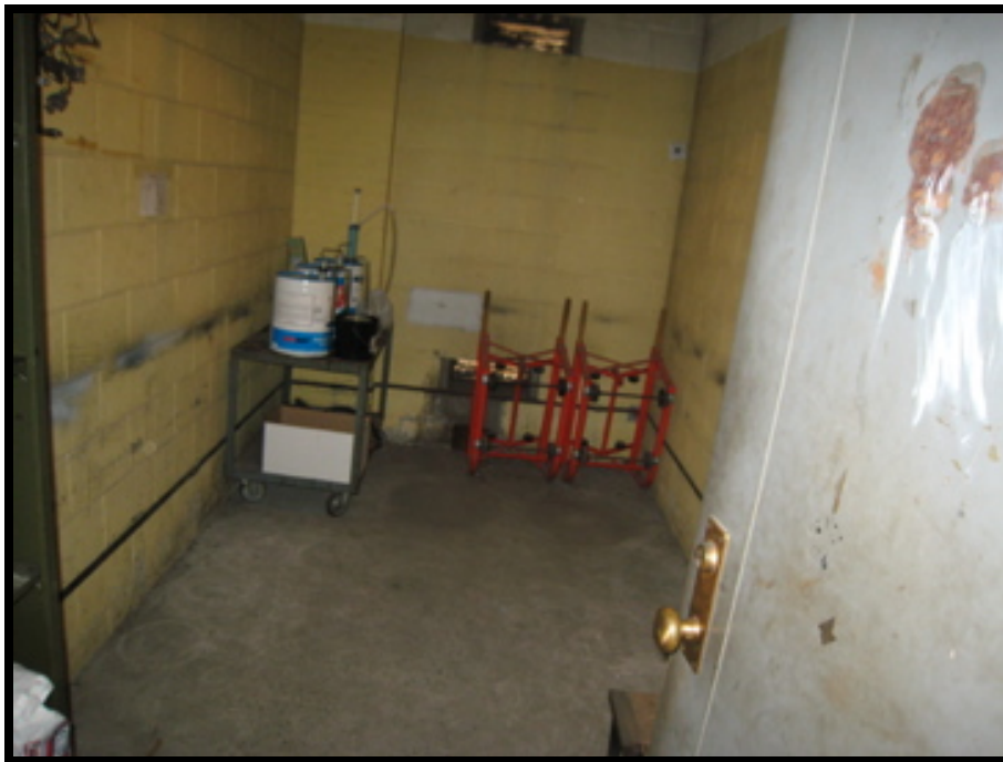
Photograph No. 8 View of Building 2 – interior – flammable storage area
