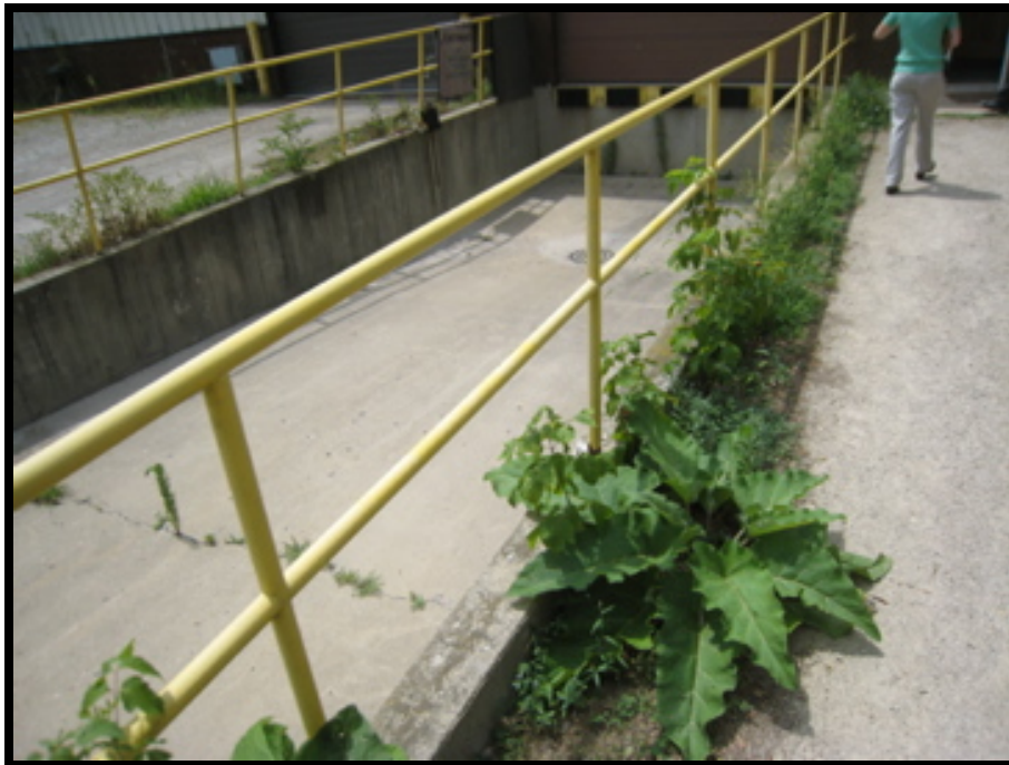
Photograph No. 17 View of Building 5 – truck well
