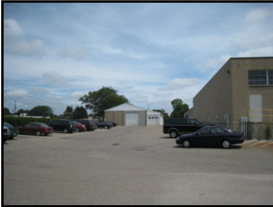
Photograph No. 1 View of subject property – Building 1 – facing east
