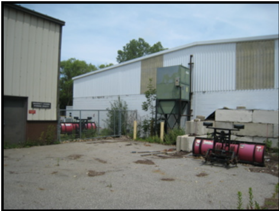
Photograph No. 16 View of subject property – Buildings 4 and 5 – facing northeast
