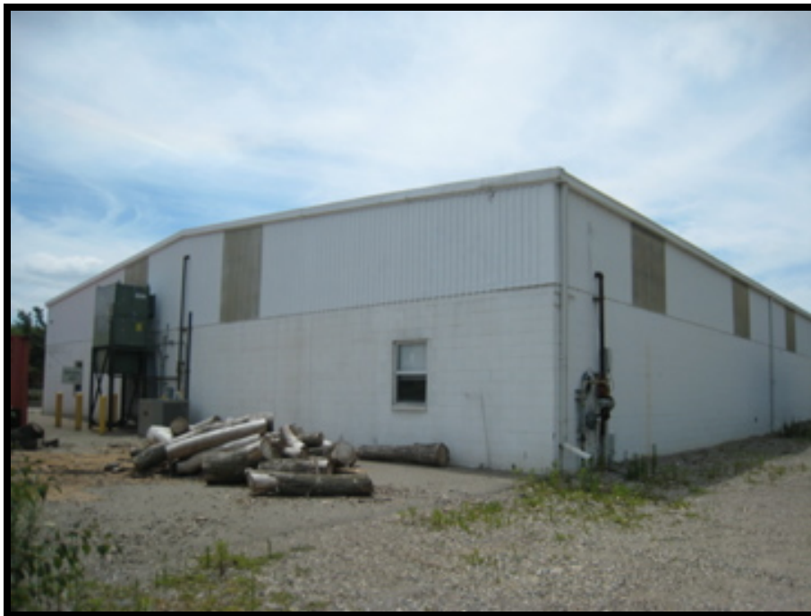
Photograph No. 14 View of subject property – Building 4 – facing southwest
