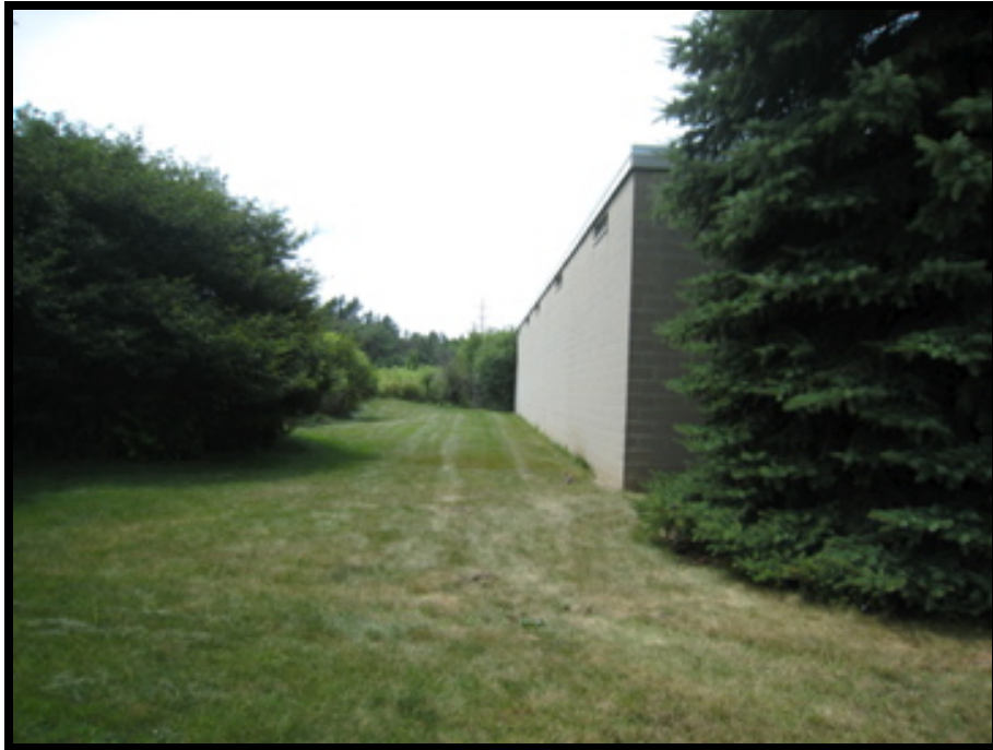
Photograph No. 11 View of subject property – Building 3 – facing west
