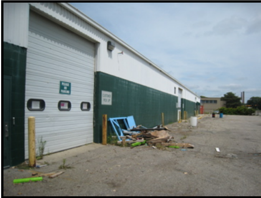
Photograph No. 13 View of subject property – Building 4 – facing east
