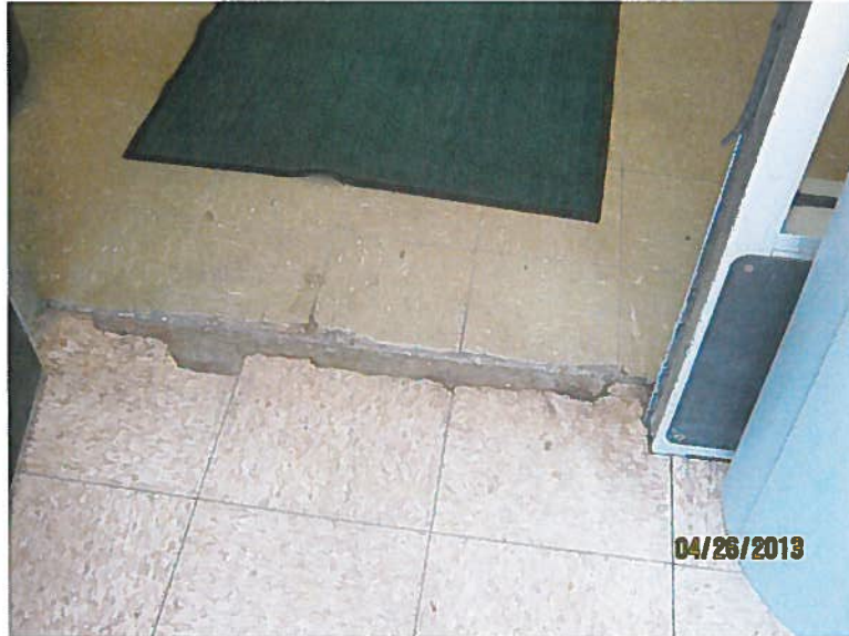
Photograph No. 1 HA-2 Amtrak Building Waiting Area 9"X9" Green Floor Tile 3% Chrysotile asbestos
