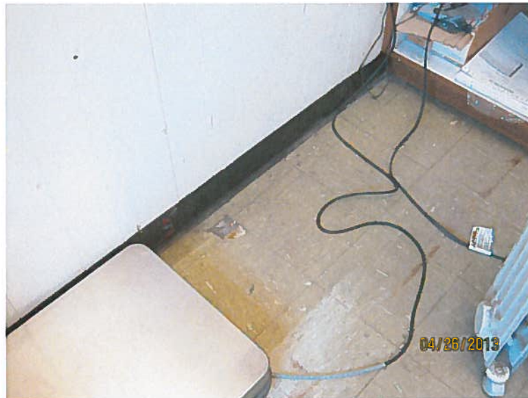
Photograph No. 2 HA-8 Amtrak Building Greyhound Office 9"X9" Gray Floor Tile 3% Chrysotile asbestos
