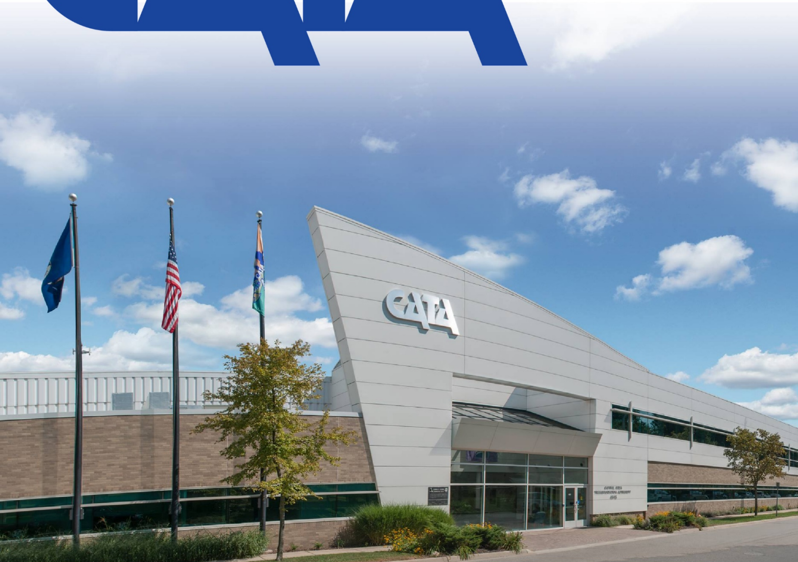
A picture of the CATA logo and below it, the CATA Administration Building.
