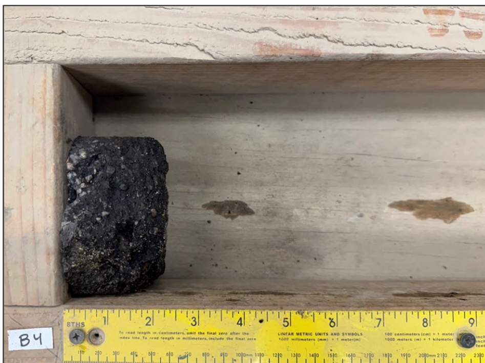
PHOTO NO. 4: Boring P4 - 2 inches of Asphalt
