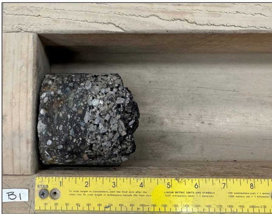
PHOTO NO. 1: Boring P1 - 4 inches of Asphalt
